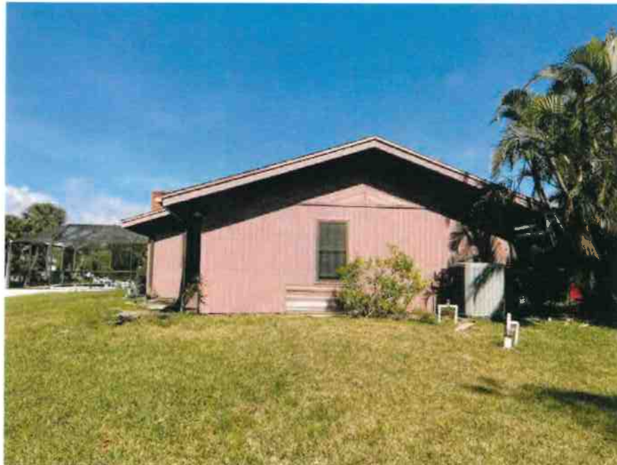
Photo Two Caption Photo Taken 02/21/2023 "Side View with A/C"
