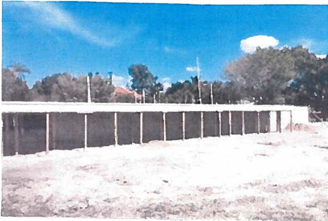
View 3: (03/01/16) South Side View
