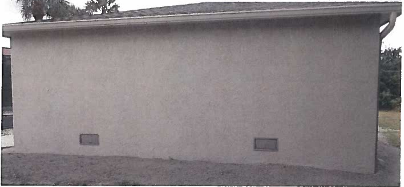
NORTH WALL - EXTERIOR
