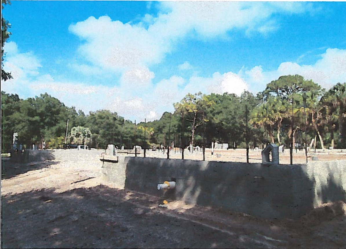
FIGURE 3: (5-23-2016) RIGHT REAR SIDE VIEW
