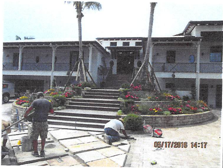
Main House Front
