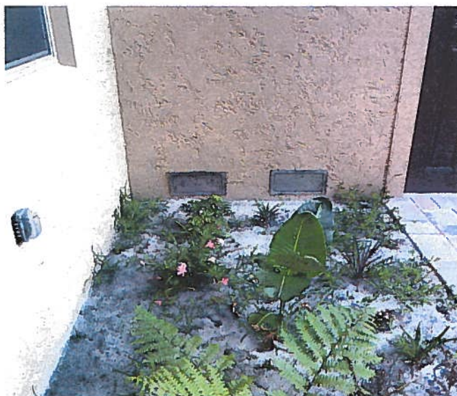
FLOOD OPENINGS Photographs Date Taken 06/13/2016
