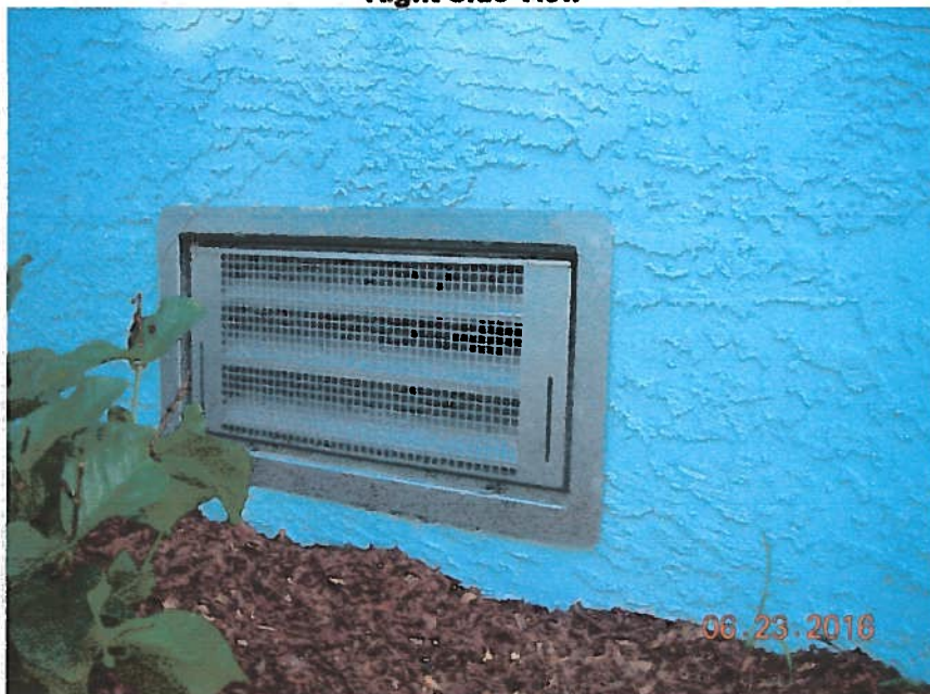
Typical Flood Vent
