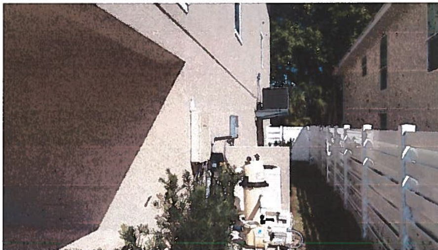
REAR-RIGHT PHOTO'S TAKEN 02/10/2016
