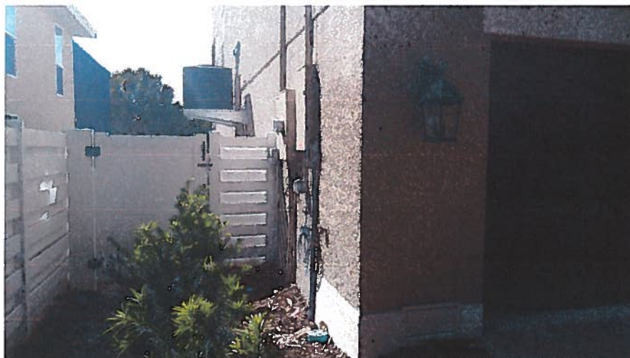
FRONT-LEFT PHOTO'S TAKEN 02/10/2016
