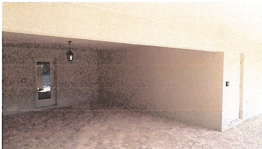
REAR-CENTER PHOTO'S TAKEN 02/10/2016
