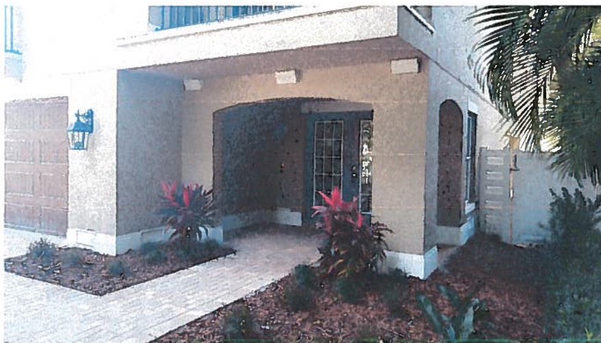
FRONT-RIGHT PHOTO'S TAKEN 02/10/2016
